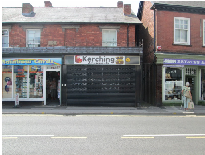
Front elevation of building
